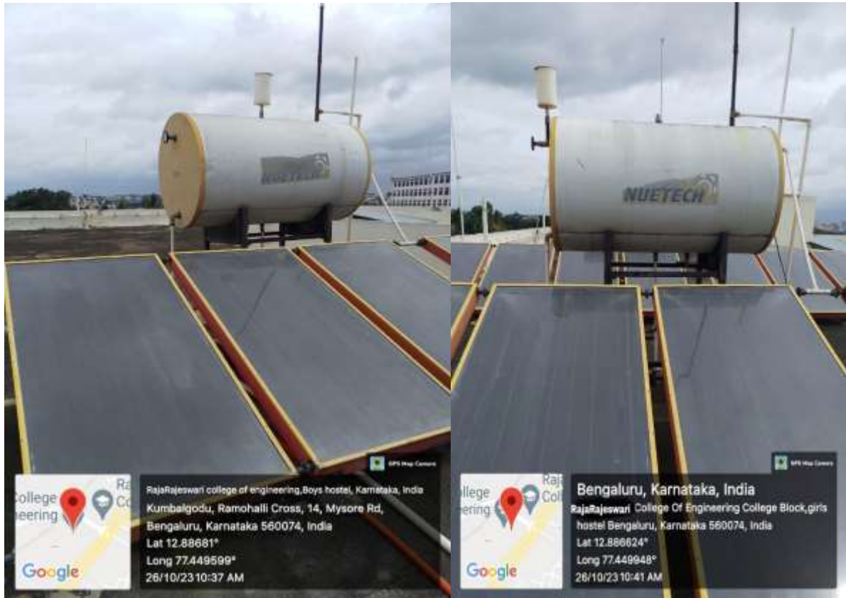
Photo.9: Cleaning solar water heating system collector panels on roof tops
