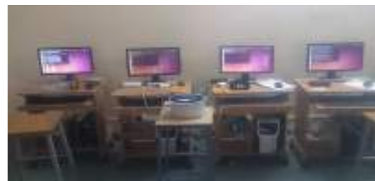
Fig 5: Multicast communication using 1KM distances of Optical cable.
