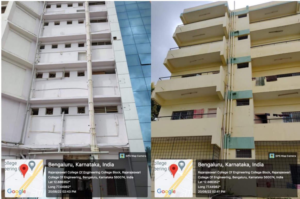
Phor.5 Duel Plumbing for Secondary Flushing
