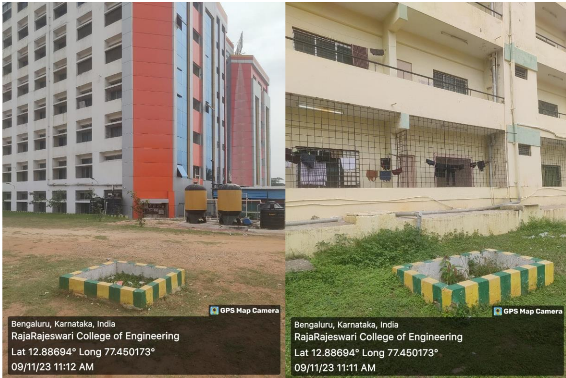
Photo.2: Borewell / Open well recharge facility inside the campus
