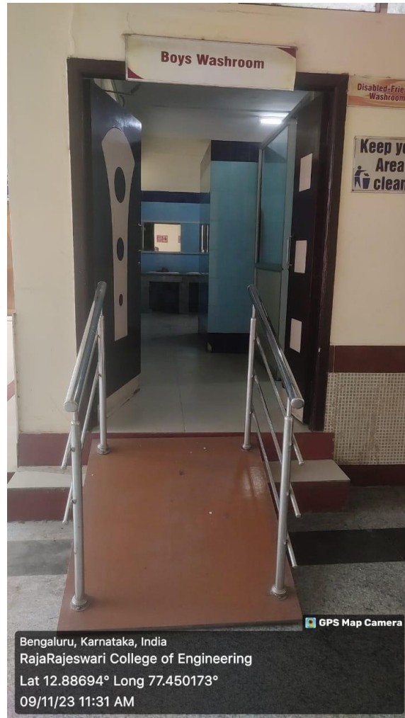
Photo.3: Disabled-friendly washrooms facility inside the college
