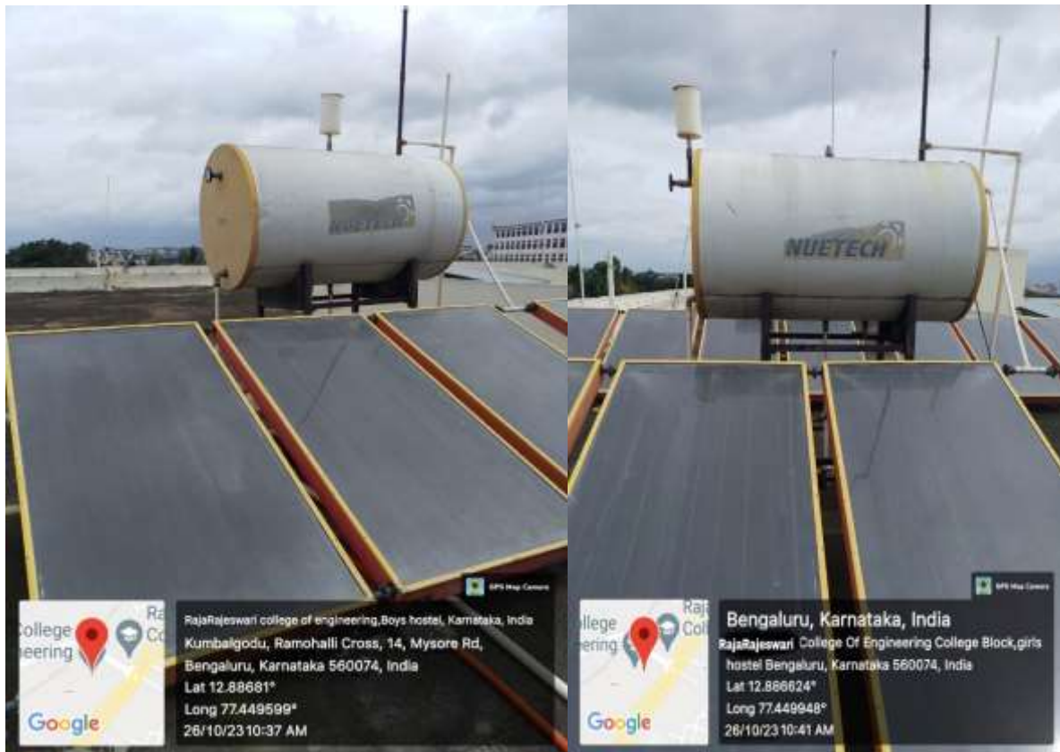
Photos 1&2: Solar water heating systems in college hostels
