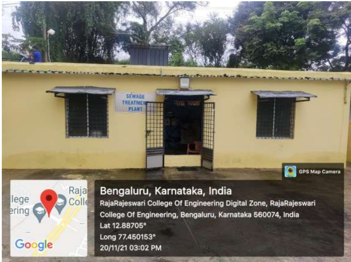
Photo.3: Sewage Treatment Plant of 100 KLD in operation at RajaRajeswari Dental College and Hospital (RRDCH)
