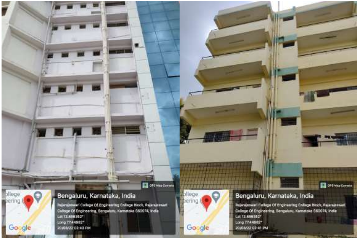
Phor.5 Duel Plumbing for Secondary Flushing
